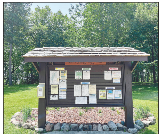
Eagle Scout Myles Jacobi coordinated the construction of this new information kiosk with a pollinator garden outside the Forest Headquarters in July.
