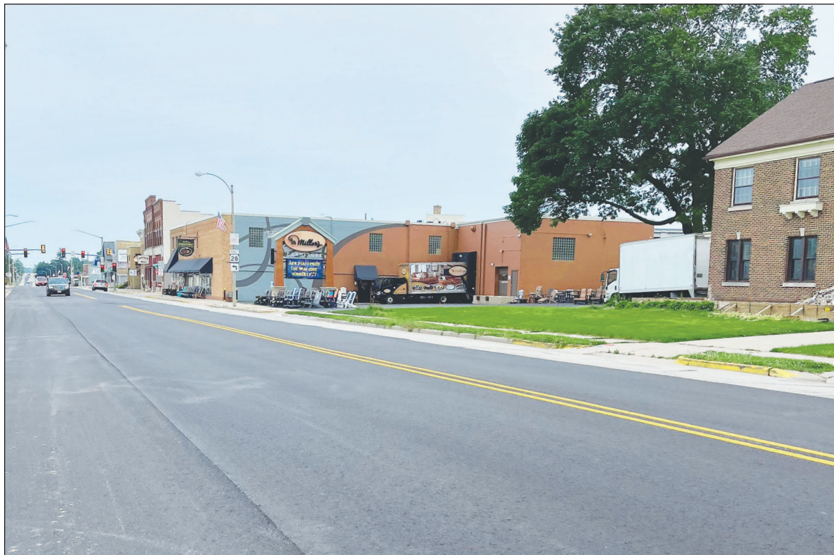
As of June 12, Fond du Lac Avenue and Main Street in Kewaskum are temporarily reopened. BREANNA RICE PHOTO
