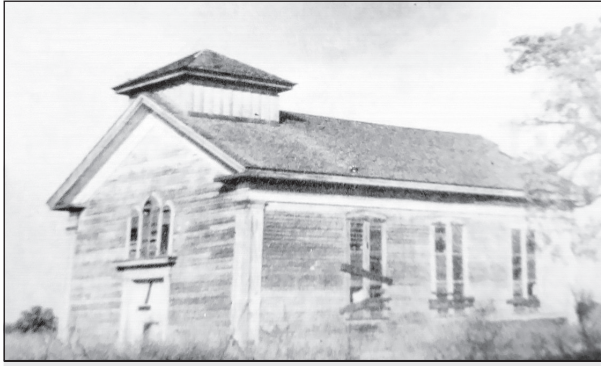
Berry Church, or the "Empire Methodist Church." According to multiple sources, the picture was labeled inaccurately elsewhere years ago. Because it was no longer used for religious services, the Hillcrest students of the 1930s used it as a place to play. According to Bob Meier, the tree on the east side of it is the large oak tree that came down recently. COURTESY PHOTO: CAROL MURPHY
