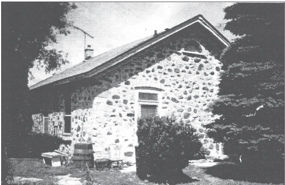
Marx School in the Town of Wayne dates back to 1851. This photo was taken in 1999.
