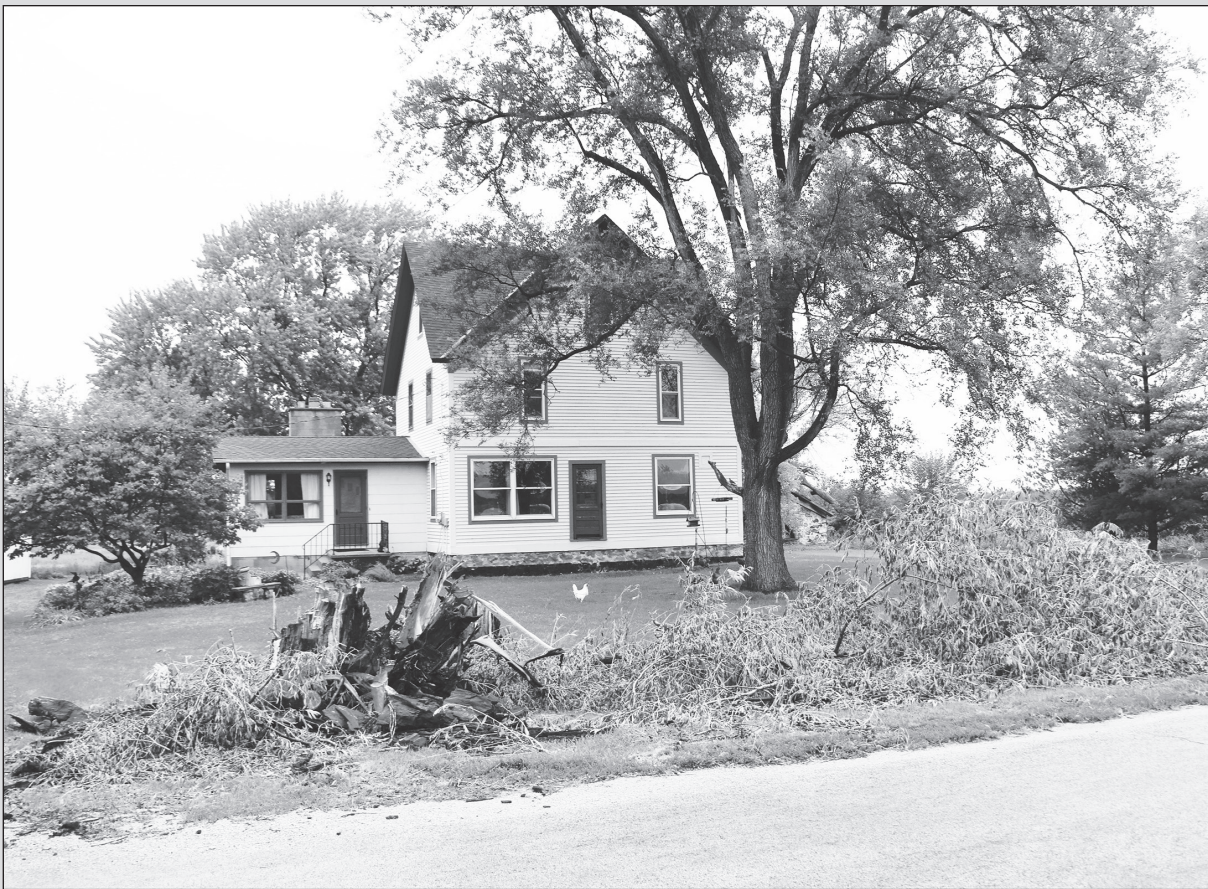
A large willow tree on Badger Road in the Town of Kewaskum is one of the casualties of a storm that came through the area on Friday, Aug. 6. Another storm knocked out power for area residents at about 4 p.m. on Sunday, Aug. 8, when utility poles on Highway H near Highland Road in the Town of Kewaskum were knocked down. PHOTO BY ANNE TRAUTNER
