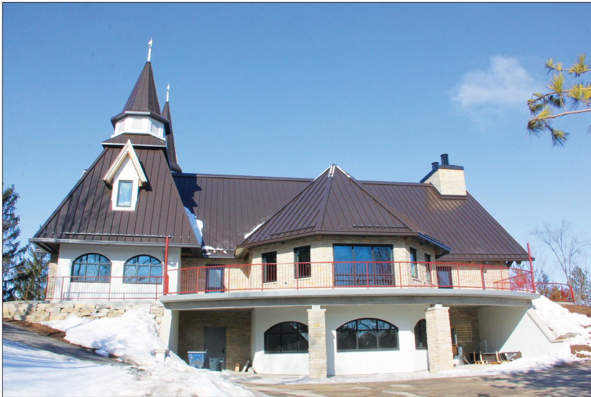
The new chapel at Camp Vista near Dundee is almost finished. The hope is to have it completed for Easter services next month. A fire in October 2018 destroyed the original chapel and construction on this new chapel started last year.
