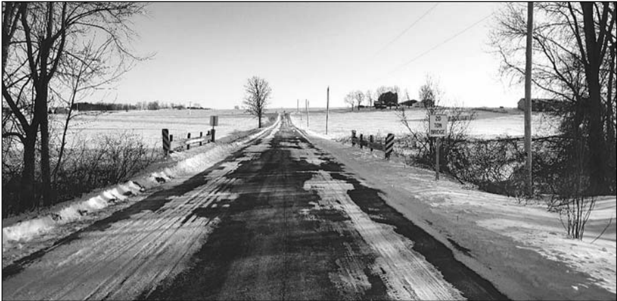
This photograph is looking south on Happy Road with the bridge crossing the Milwaukee River tributary. Underneath the old bridge was Prindle Hole, which was a great place for youngsters to swim in the 1940s.
