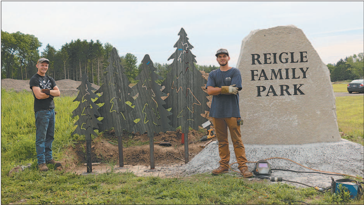
Myles Ottery and Macaulay Derge of Dean Derge Ornamental Ironworks stand beside the metal trees they installed as part of the Reigle Family Park sign. Made of Corten steel, the metal trees will rust to provide a contrasting color with the gray stone.
