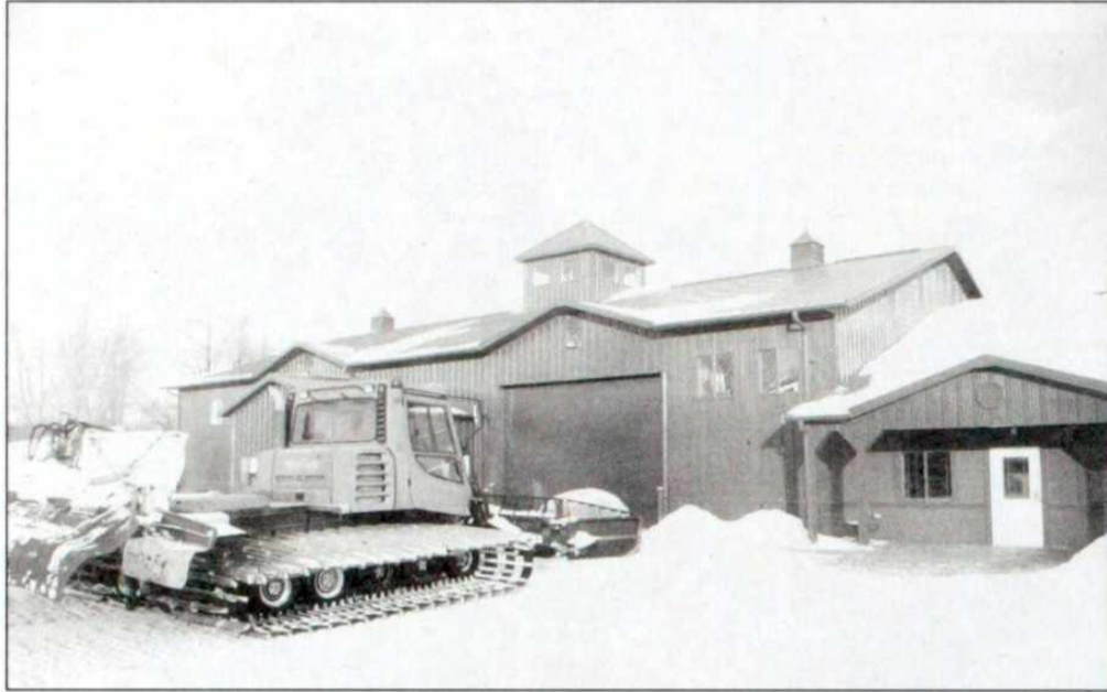
Sunburst constructed the new storage building shown above after a fire last year destroyed the former structure and some of the equipment inside.
