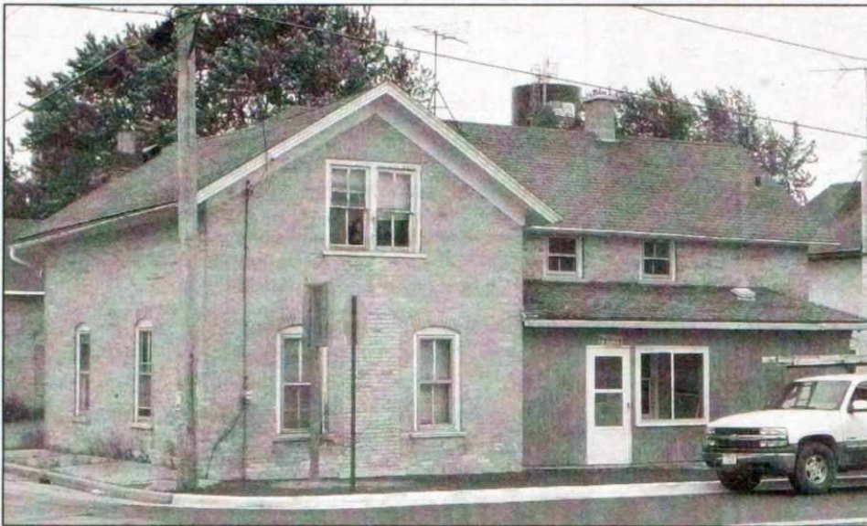
This home at the corner of Highways H and W in the town of Wayne is being considered for a vision triangle by The Washington County Highway Department.
