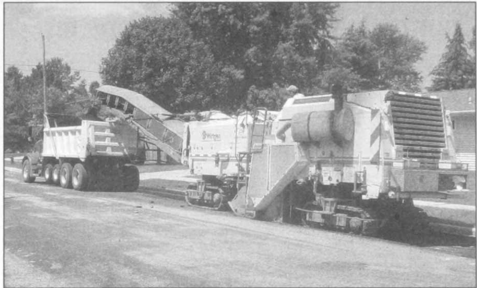
A Payne and Dolan milling machine shoots milled asphalt into a dumptruck from Dundee Sand and Gravel Tuesday on Lin-de-Lane in Kewaskum.
