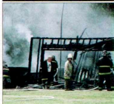
Two-alarm fire in Kohlsville/ Home partially destroyed
