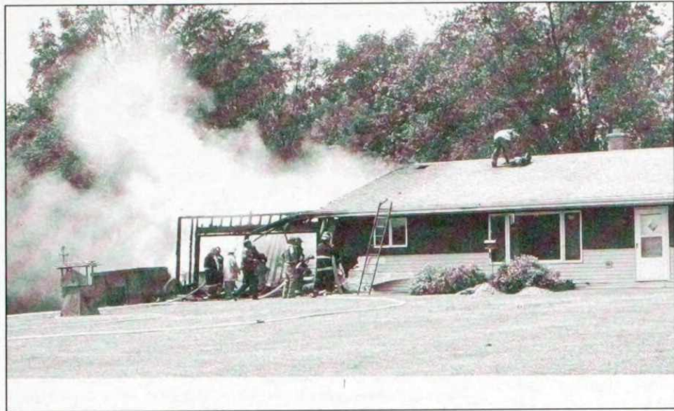
Kohlsville firefighters work at extinguishing a fire at the Armand Mertz home on Thursday, July 6.
