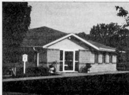
Maple Dale Manor of Kewaskum II 14-Unit CBRF
