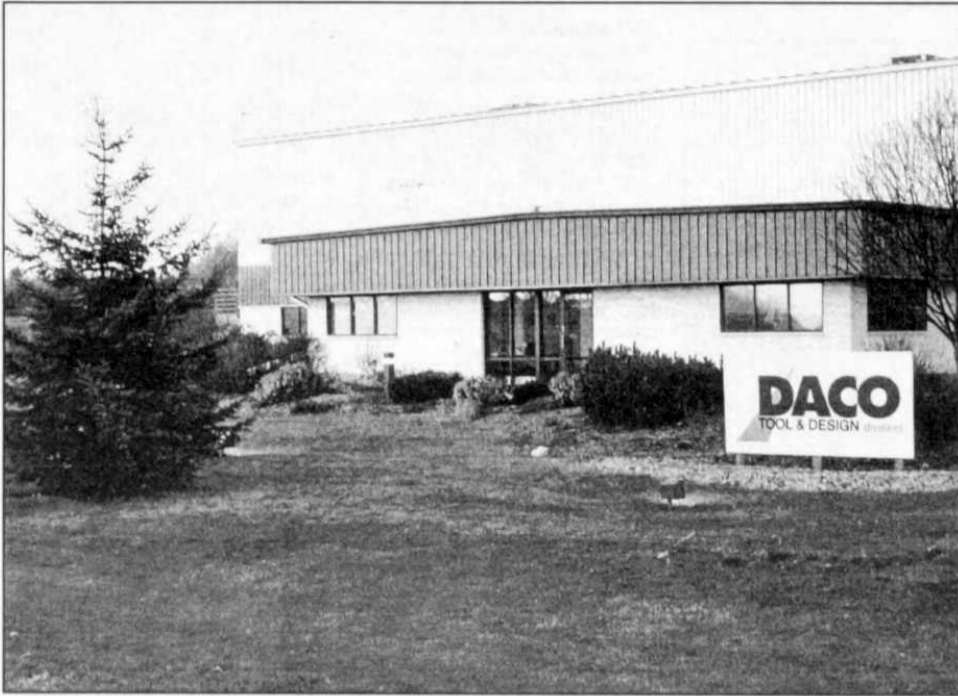
DACO Tool and Design is located in the Village of Kewaskum's new industrial park on USH 45. The firm intends to proceed with a 53,000 square foot addition.
