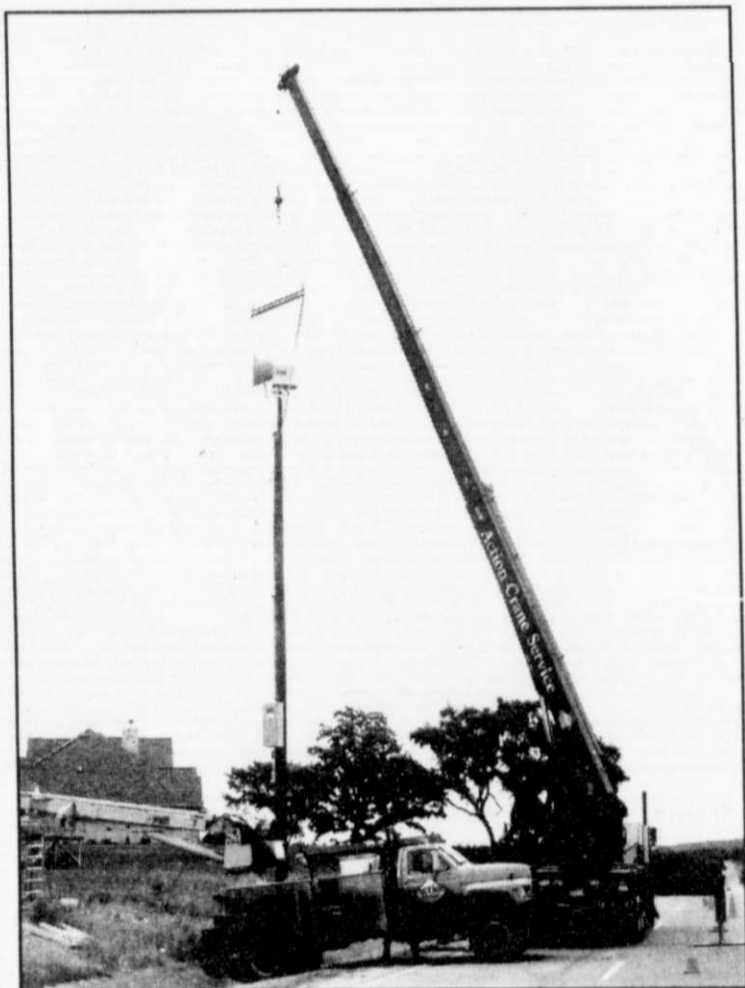
Workers from Action Electric install the latest emergency siren in the village at CTH H west and Kettleview Drive.
