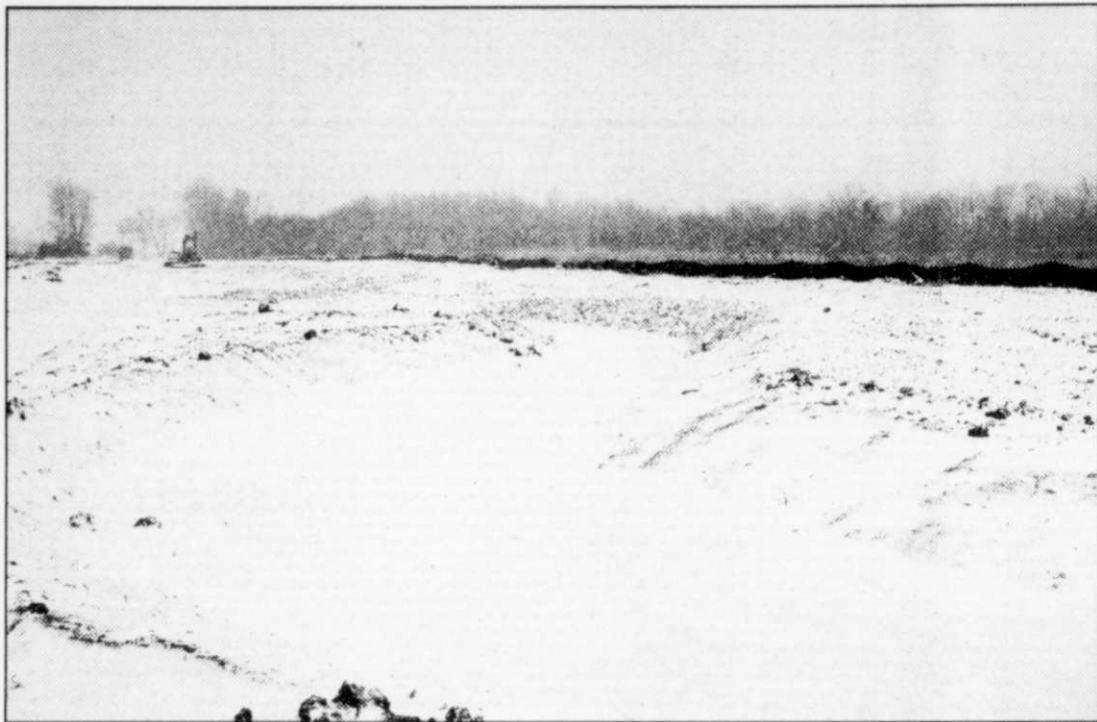
Shown above is a view of the stream being constructed along USH 45.
