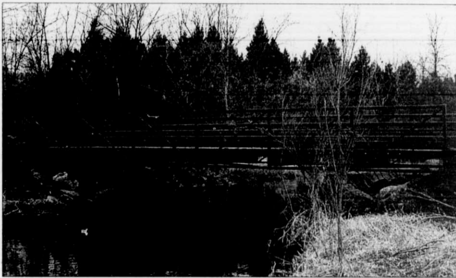
A view of the installed snowmobile bridge over the east branch of the Milwaukee River. Submitted Photo
