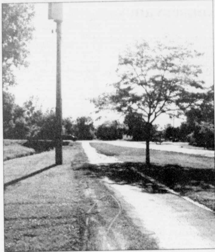
The skate path project was completed this week in front of the fire station. The trail starts in Riverhill Park by the dam and ends at Hwy 45.
