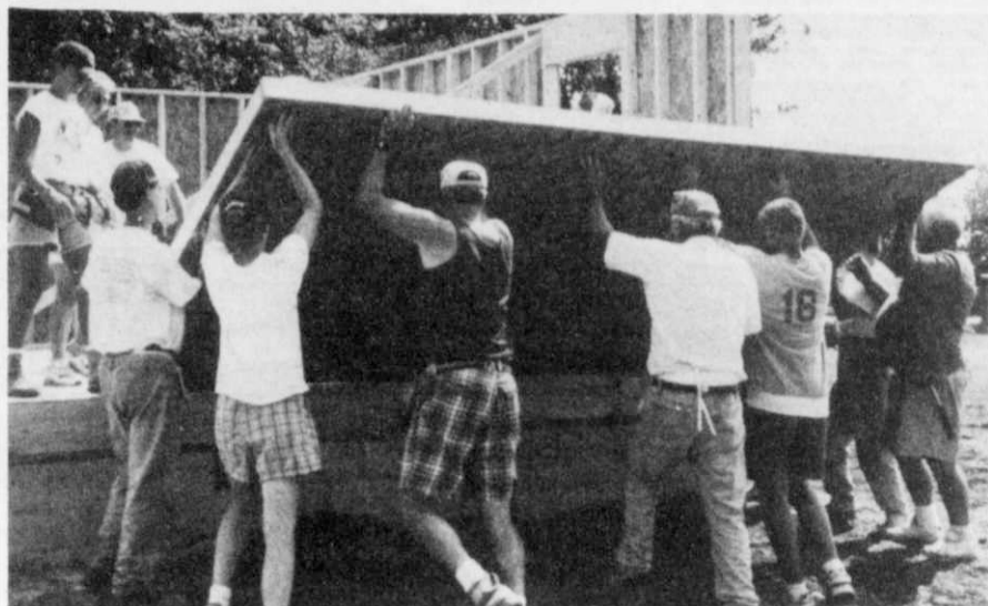
Exterior walls get the attention of many Peace Church volunteers.
