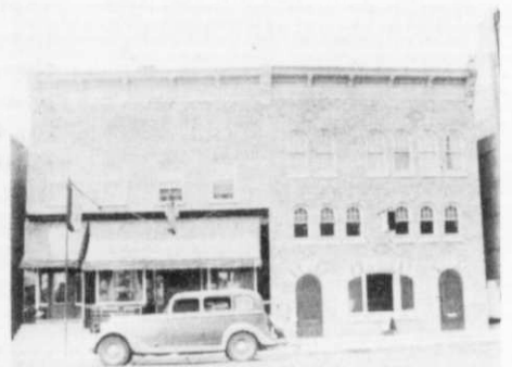
Later photo of remodeled building
