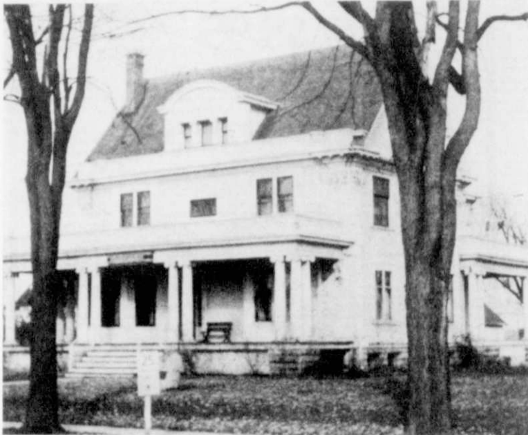
The former Henry J. Lay home was purchased by the American Legion in 1945. Pictured above is the building with all three levels intact.
