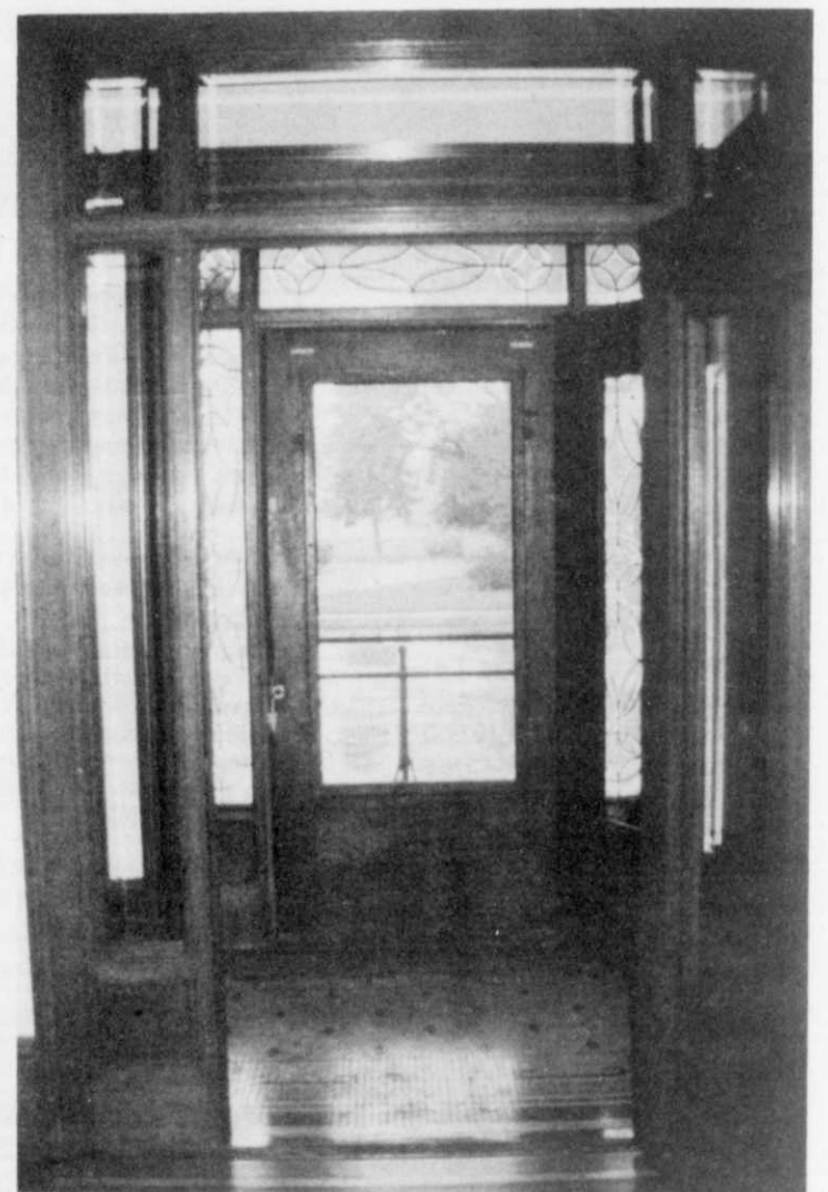
The original entranceway boasts carved oak woodwork, beveled and leaded glass, and an inlaid tile floor.
