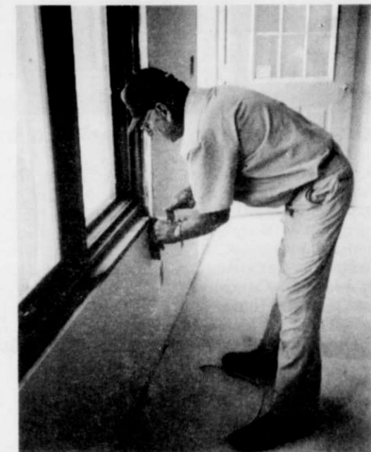
Clayton Stautz does finish work at the Moran site.
