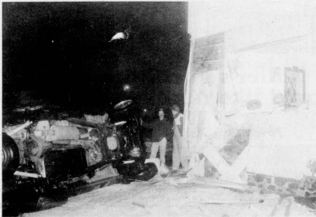
The overturned vehicle which ran into the Family Hair Salon building on Main Street Wednesday evening is shown to the left of the photo, along with the damage done to the exterior of the beauty shop.
