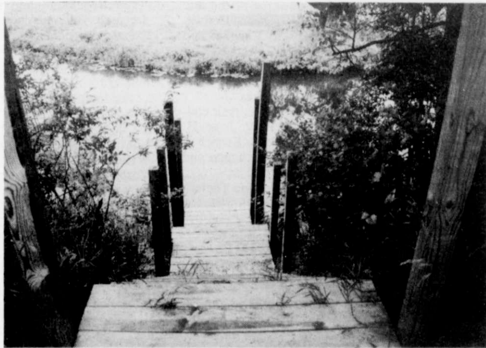
Steps leading down to the river were built by the high school construction class and will be finished sometime this school year.
