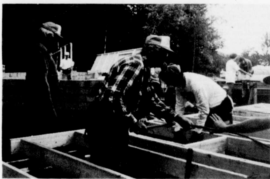
Some built sidewalls while the foundation block was laid.
