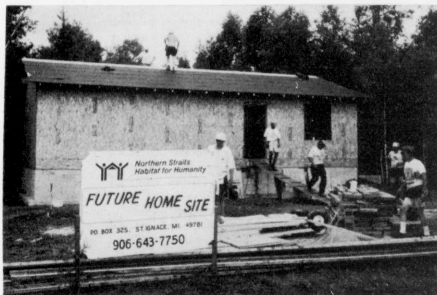
The house nears its completion at the end of day five.
