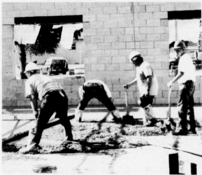
Concrete slabs were poured in the interior of the front addition of the high school.
