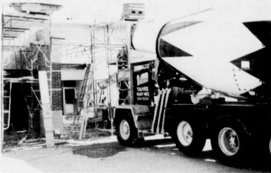
Pouring concrete in the front of the school.
