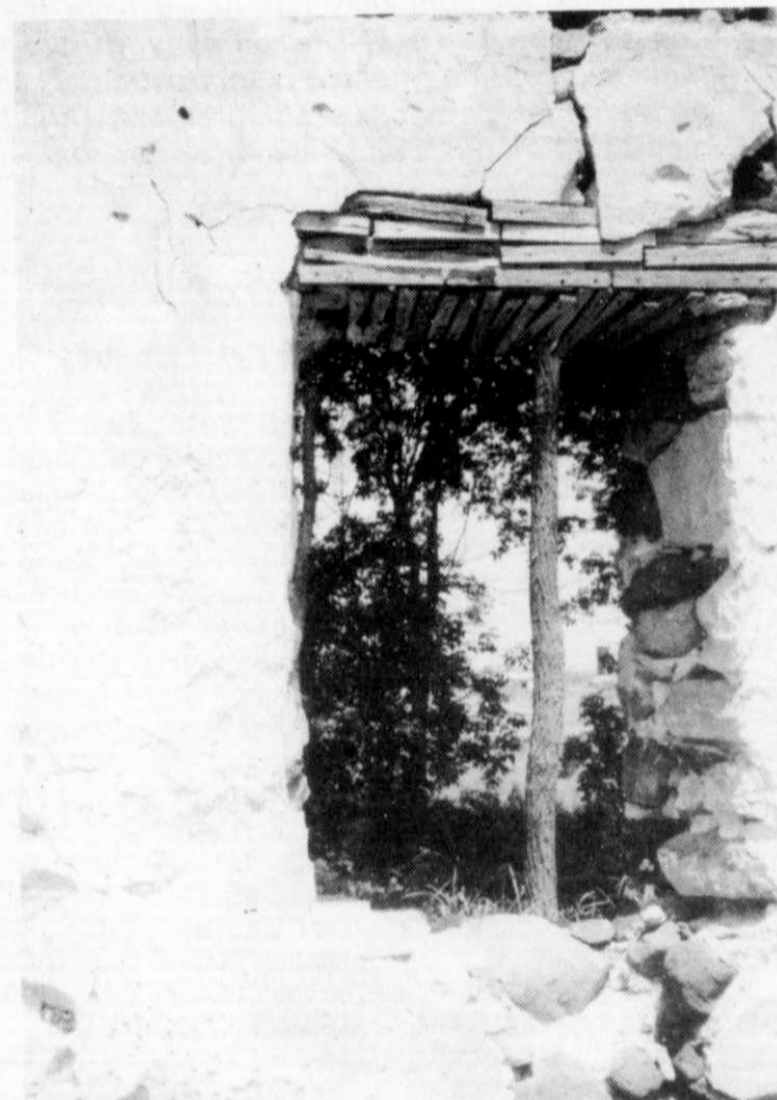
Deterioration of the 18 inch thick stone walls is evident from the back of the building.
