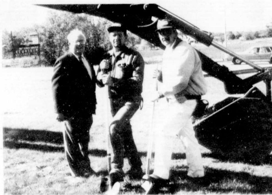
Groundbreaking ceremonies for FUMMC's balancing plant included (L to R) Don Uelman, general manager of FUMMC, Tyrone Arneson, Kewaskum plant manager, and Steve Joas, district 6 director of FUMMC, and also a producers.
