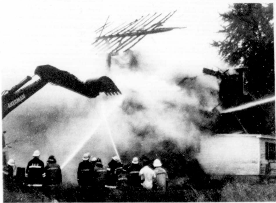
Members of the Kewaskum and Boltonville Fire Departments, pictured above, and the Kewaskum Department's Tele Squirt pumper to the right of the photo, continued to pour water on the smoldering hay and the backhoe being used to pull the hay out of the barn.
