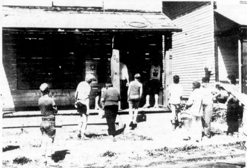
Inspection of Kingsley Street house by the Harmonia gang.
