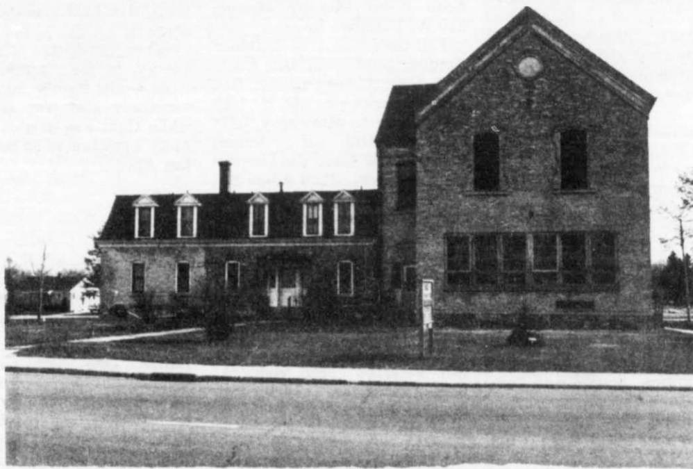
The original two-story school and convent which stood along Main Street for over 100 years, has been torn down. The only evidence of their existence are pallets of bricks which are for sale by Holy Trinity parish.
