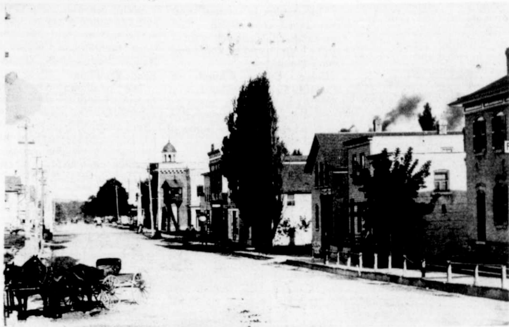
The above oldie from 1905 shows Main Street in Kewaskum. Note the crossing gate tower at the railroad site and the horse hitching rails.
