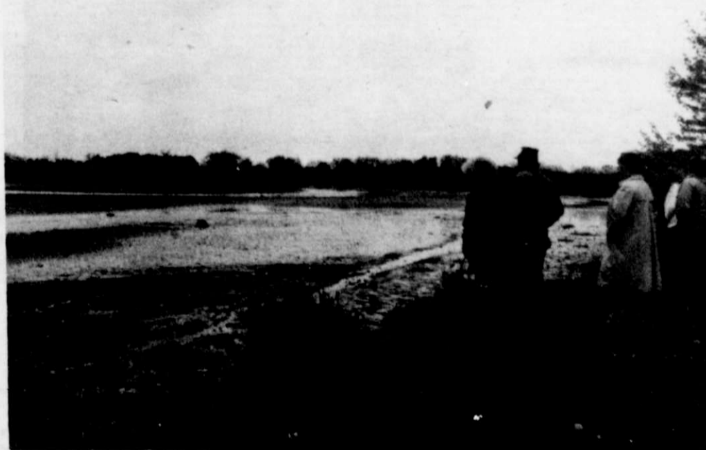
The Watershed Tour viewed the drawn down impoundment area behind the West Bend Woolen Mills dam. There is presently a controversy over whether or not the dam should be removed or replaced. Besides the highly contaminated sediment in the basin, there are 3 landfills along its banks which may have water back charging into them which could again pollute any cleanup measures taken in the near future. One of the DNR's options is to remove the dam and fill in the impoundment making it a grass area. Property owners along the dam area are opposing that action.
