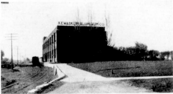
This is the original building of the Kewaskum Aluminum Company plant which had its humble beginning in 1919 and was completed in 1920. It was started by Adolph Rosenheimer, Sr. Following his death in 1943 an eventual decision was made to sell the company. It was sold in 1945 to James O. Reigle of Massillon, Ohio, and the name was changed to Kewaskum Utensil Company, with J. O. Reigle as its general manager and president. In 1951 the company's name was again changed to Regal Ware, Inc. Since purchased by Reigle, the company has greatly expanded. (Photo submitted by Tiny Terlinden)
