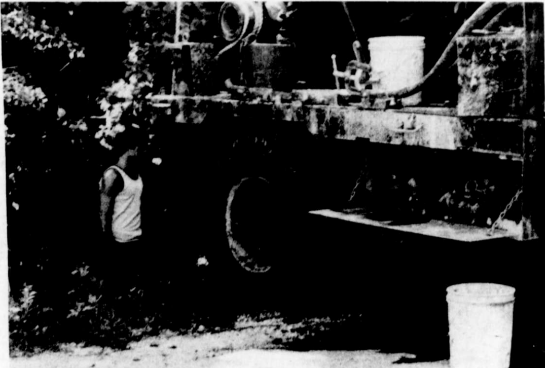
Workers from S.T.S. Consultants drilling the third of four test wells in and around the Farmington landfill site. The drilling was conducted to determine if seepage from the site is causing pollution of the nearby groundwater. (Chuck Voge photo)
