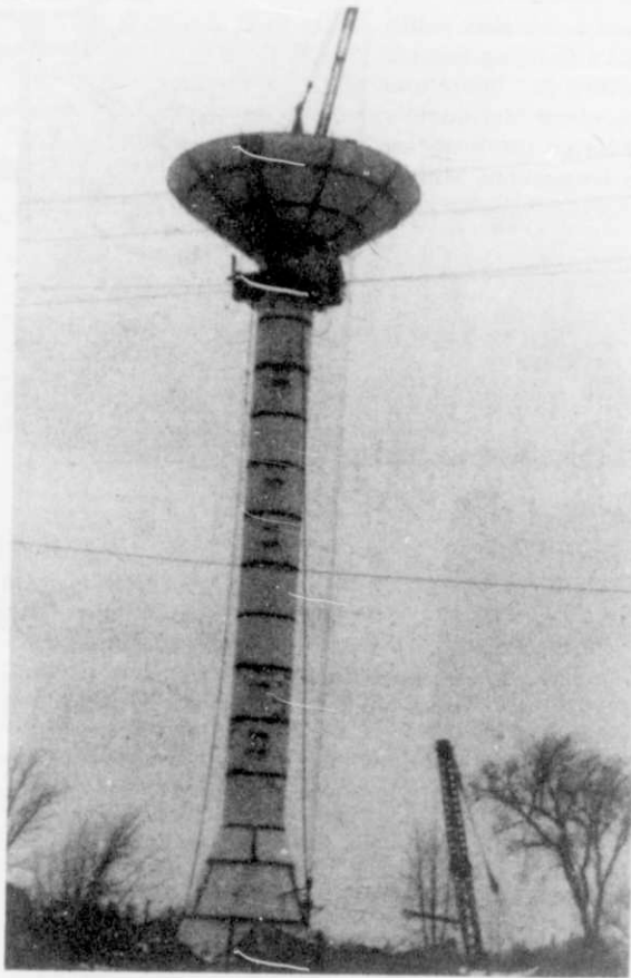
The pedestal base ready for the side sections.
