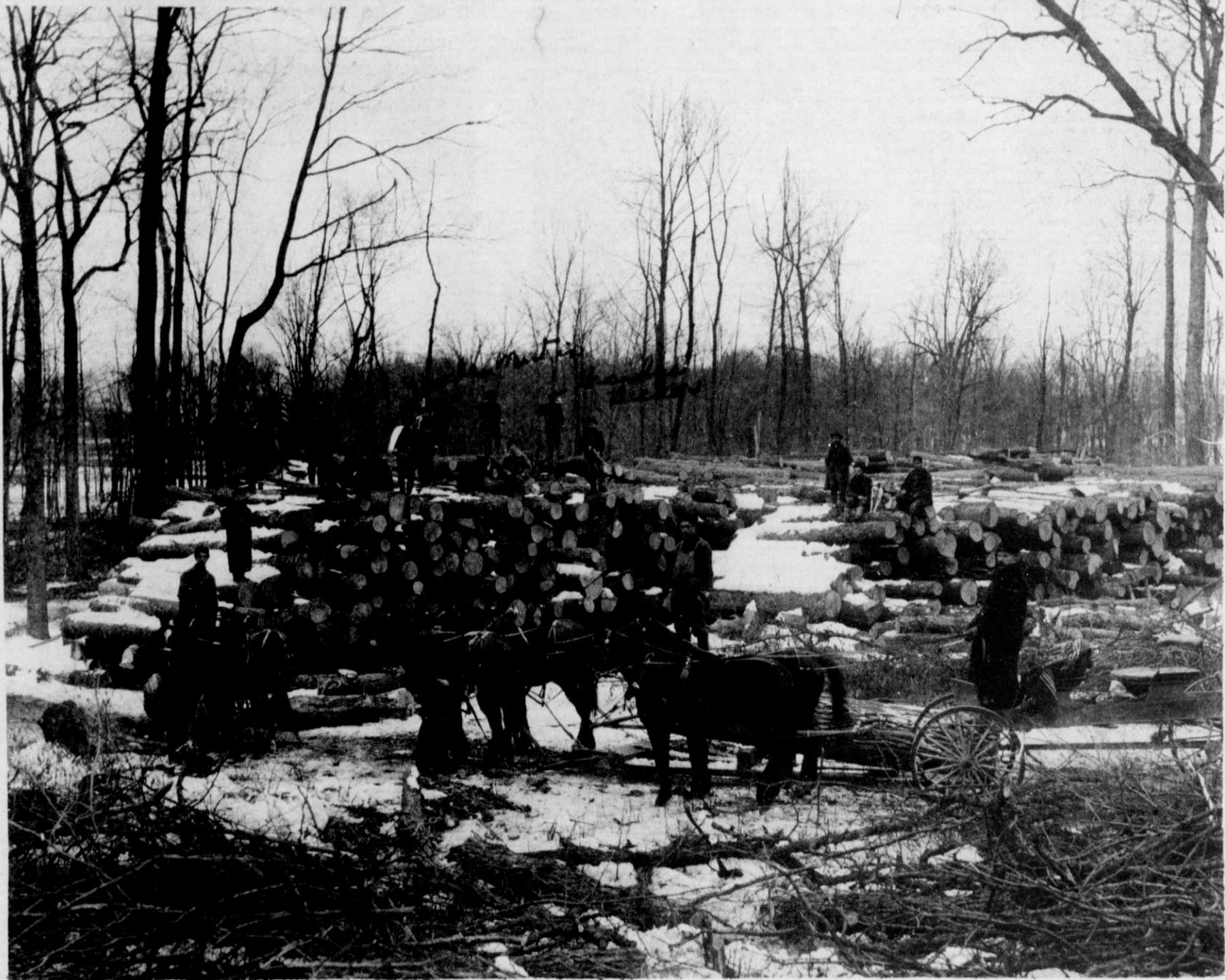
Here is an old photo, taken way back in 1886, showing a land clearing and logging operation somewhere north of Kewaskum. Two of the men on the log
