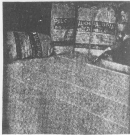
Pal-O-Pak Insulation spread between the joists under an attic floor.
