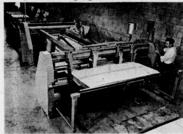
Badger Packaging Corporation of 300 per minute. This machine of Kewaskum has installed a new not only adds to Badger Packag-Swedish automatic folder gluer ing's capacity but will make a The machine is capable of folding, more exacting box for their many squaring, glueing, and automatic-customers. ally counting cartons at the rate
