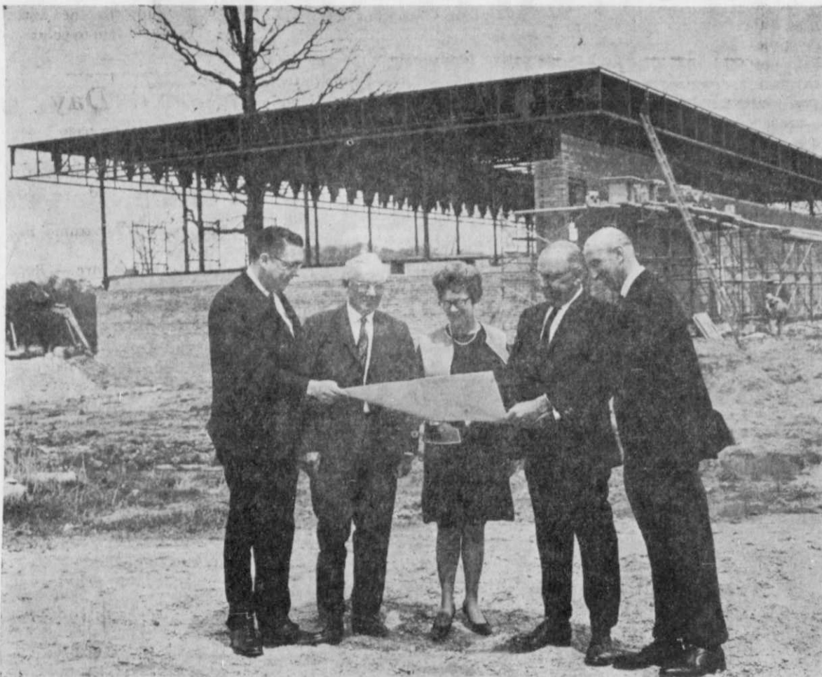
(Story on page 1) Checking the floor plan on the new office unit of Regal's Administrative Center are from left to right: James D. Reigle, presi-
