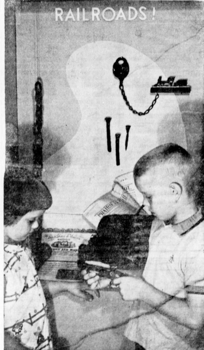
In the decade before the Civil War railroads penetrated the Wisconsin wilderness and a route to market was opened for the products of the frontier farms. This year's Historymobile closes as the secession of South Carolina from the union heralded the approach of the Civil War.
