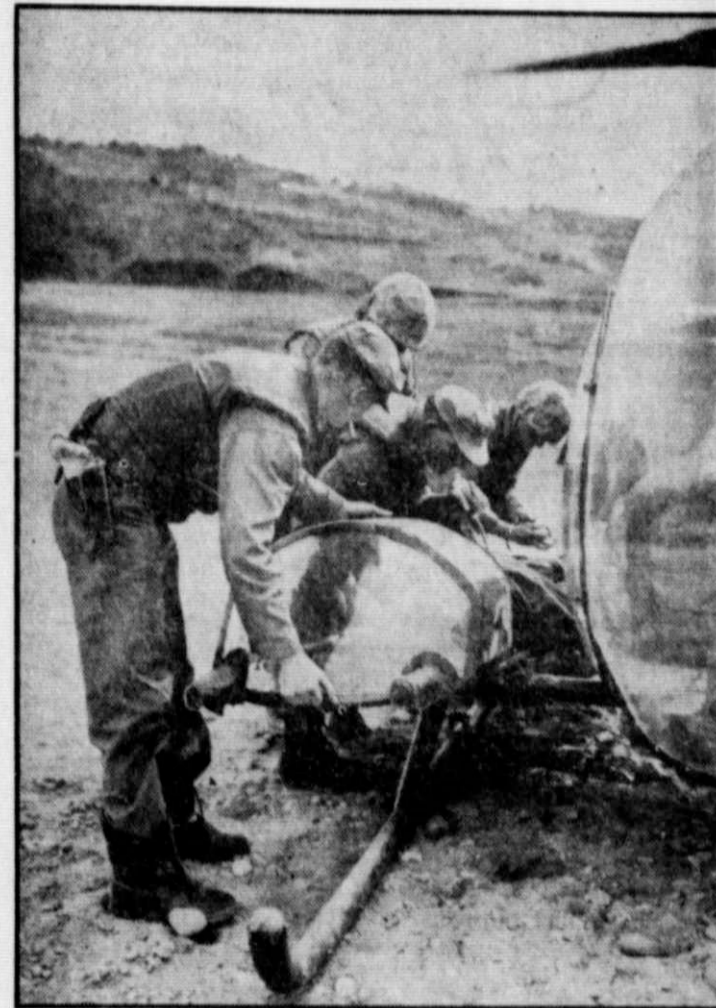
AERIAL SIDE CAR —Covered with a plastic hood, this wounded G.I. is being readied for a trip to a rear area somewhere in Korea. Stretchers fit into specially constructed side attachments of the helicopter and ride the air comfortably. This casualty victim is receiving blood plasma before making the trip.
