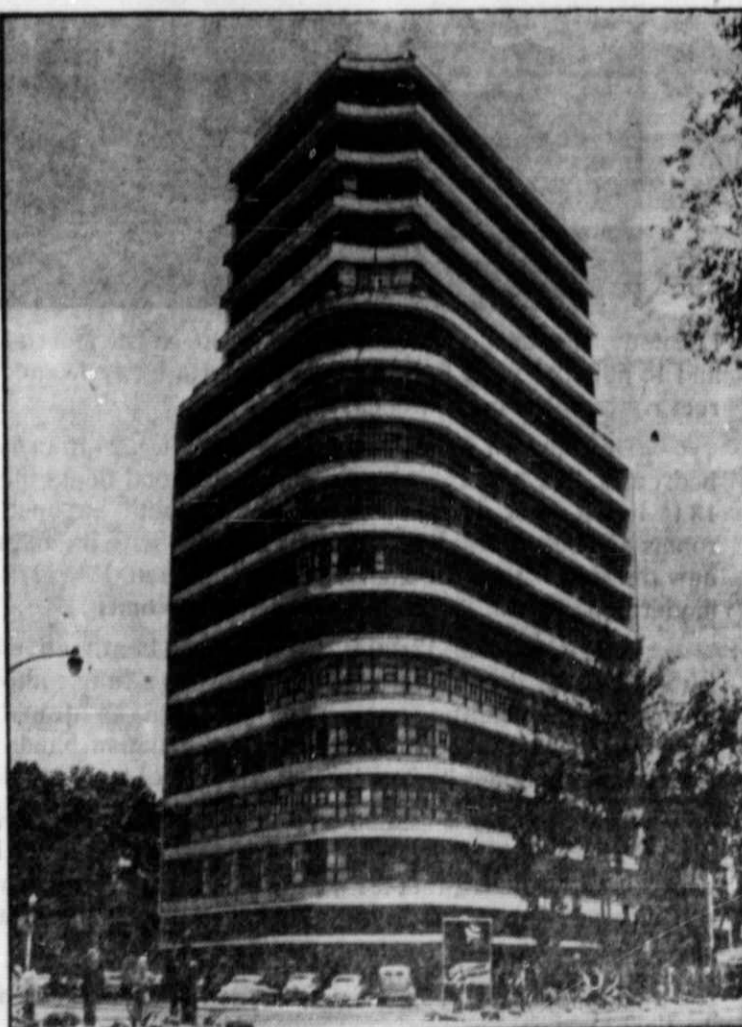
BIGGER AND BETTER —Previously scattered in four different buildings, the U. S. Embassy in Mexico now occupies this modern 17-story structure on the Paseo de la Reforma in Mexico City. The only U. S. Embassy in the world larger than this one is in England.
