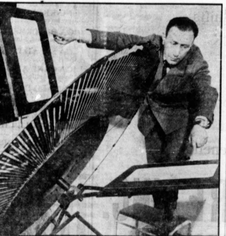
TRI-DIMENSIONAL WHEEL —Something new in the projection of three-dimensional movies has been invented by Alberto and Adriano Betti. Instead of giving spectators glasses, the Roman twins synchronize a projector with this revolving glass disc which has alternating mirrors and transparent segments. Two images are projected through the disc, one reaching the viewing screen, left, while the second is reflected by the mirrors to another screen, right, and from this back to the viewing screen, giving a third dimensional appearance to the movie.
