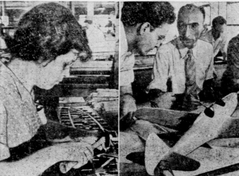
A BORN RIBBER . . . Ribbing is the assembling of the framework of the wings. Vilda E. Seibert is engaged in that task here. The wings of the plane are covered with plywood after this job is completed. BRAIN DEPT. . . . Before you can start to build an airplane there are scores of things you must know about aero dynamics. Here are two project engineers dopping out stress, weights, etc.
