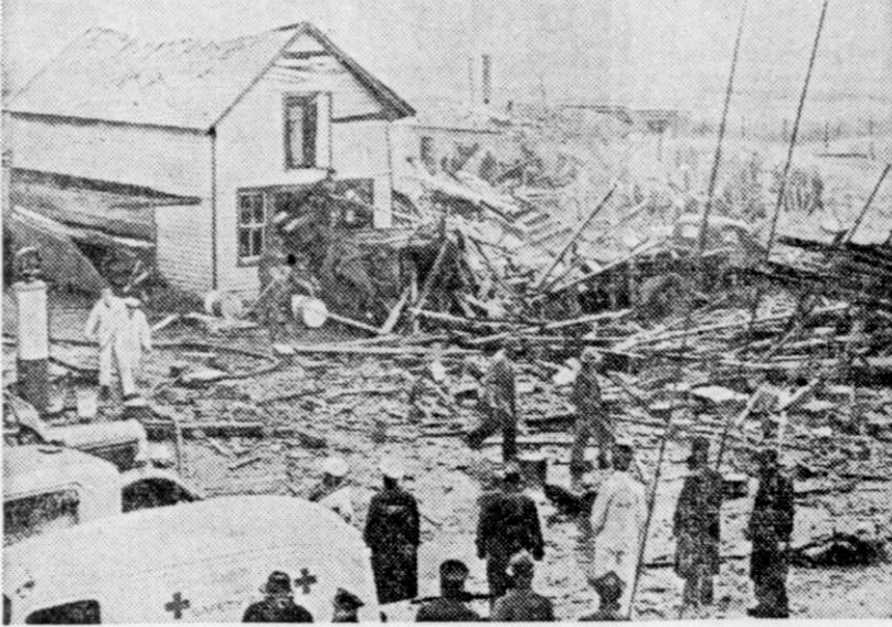
WOODBRIDGE, N. J.—This scene of desolation met the eye after a terrifying blast leveled the United Railway and Signal Co. here, killing nine persons and injuring 33. Though the plant made torpedo signals for railroads, it was said to be working on a device of "great importance" to the army and navy. (For news of other powder plant blasts see "DEFENSE: Supplies.")
