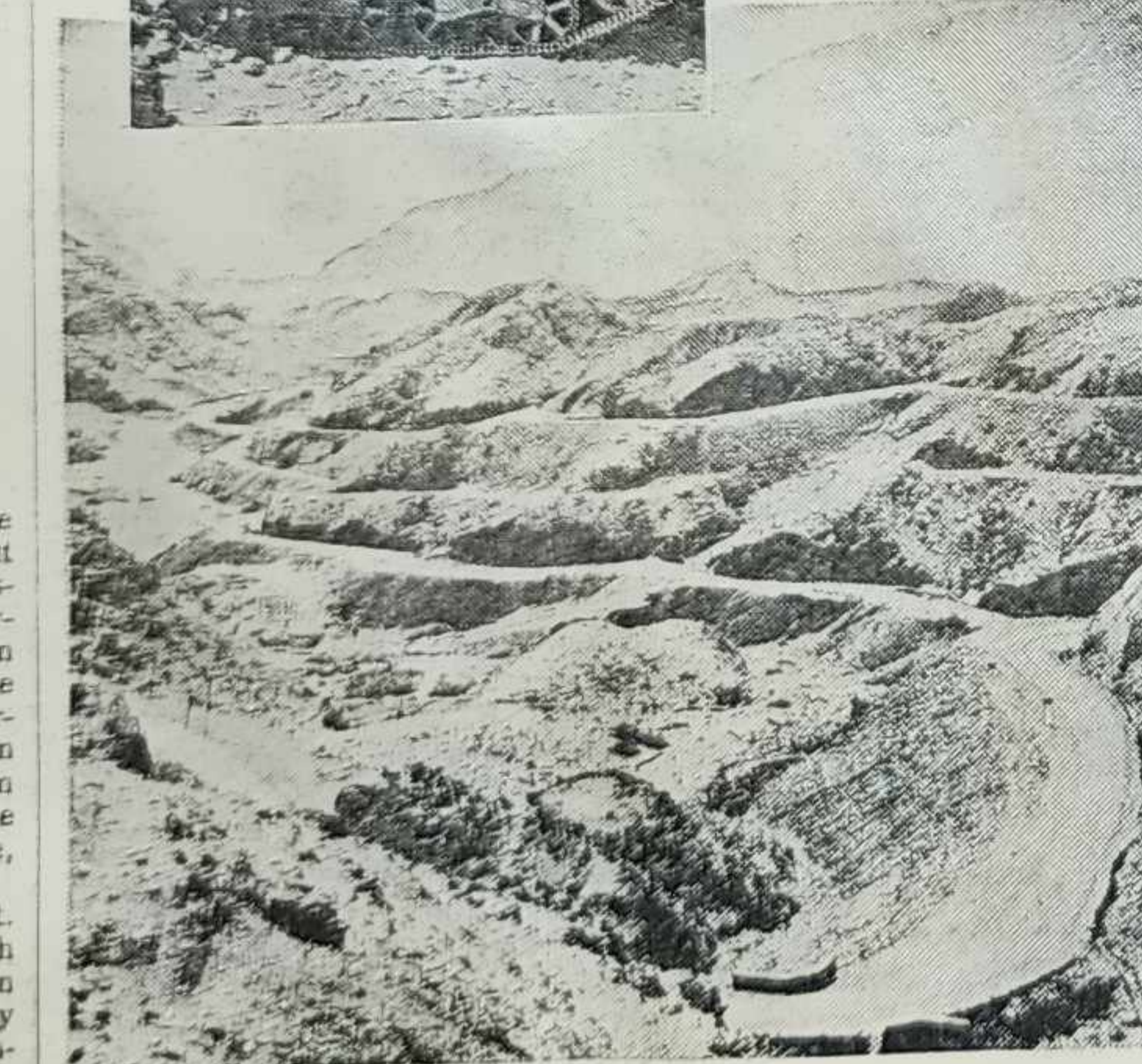
Above is the Khyber pass itself, showing the trouble confronting an invader aiming to penetrate it. A remarkable serpentine road winds through the narrow defile for 33 miles. There is also a railroad, completed in 1925. It is a marvel of engineering, 26 miles long with 34 tunnels and 92 bridges and culverts. Each station is a miniature fort.
