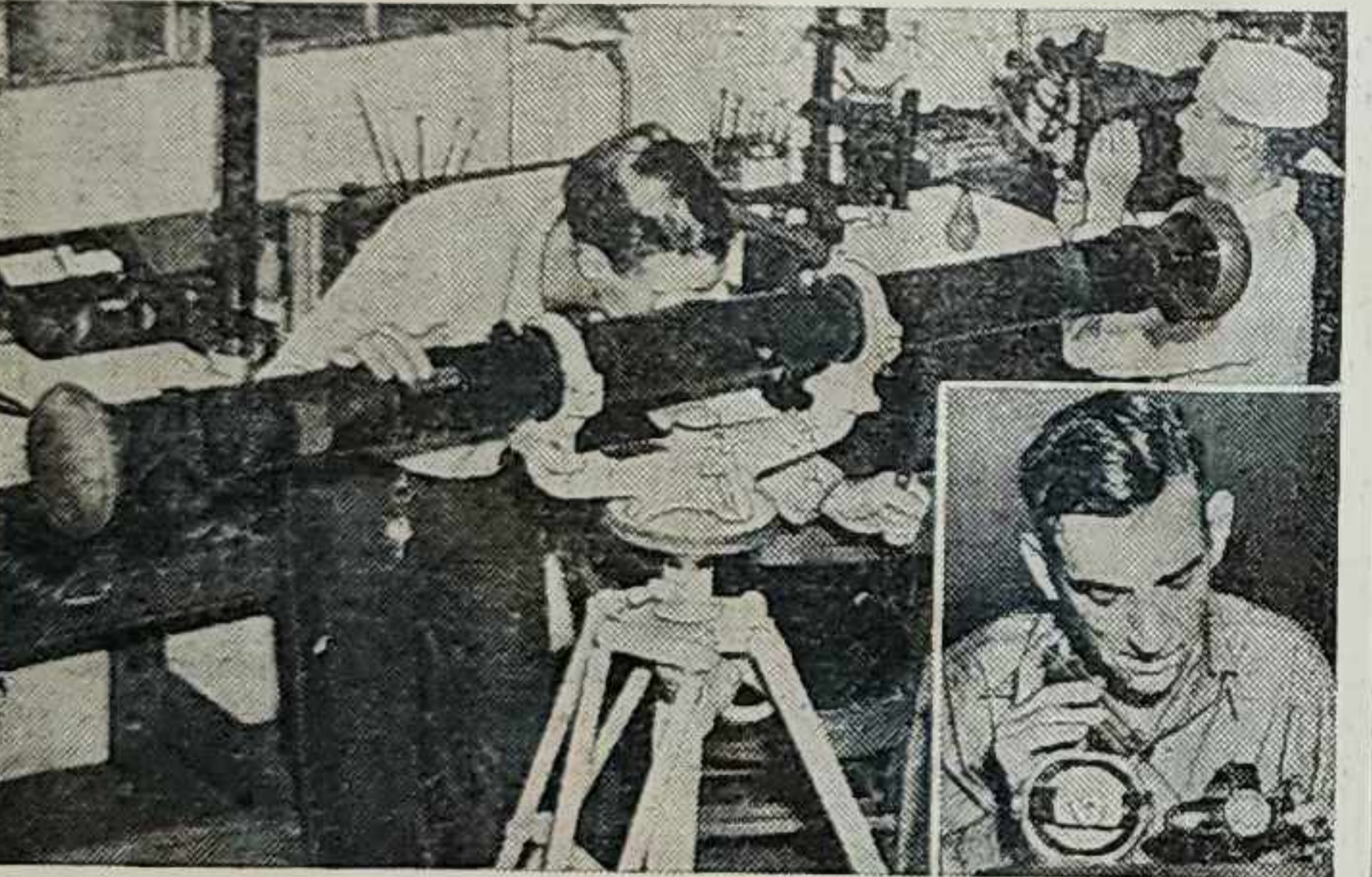
A range finder is given final inspection, while in the background another naval optical shop expert checks a sextant. Inset: Seaman working on a gyroscope, which governs path of a torpedo after it has been fired at a naval objective.
