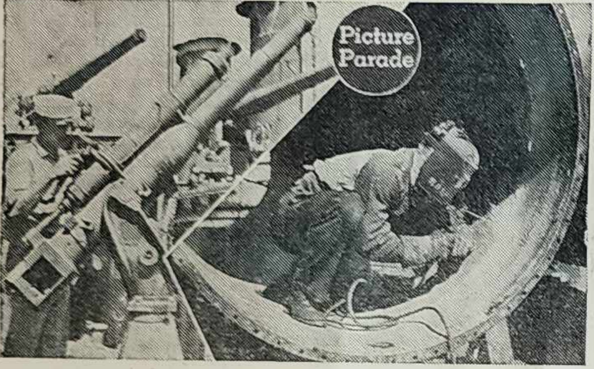
Left: A seaman chips preservative red lead from a three-inch anti-aircraft gun aboard one of these recommissioned destroyers. Right: A welder works on one of the huge smoke stacks removed from the USS Williams.
