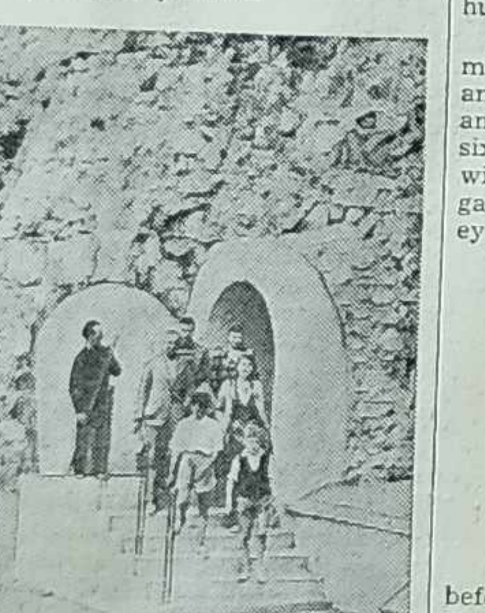
FOR HOSPITALS—Here is harbor entrance to Ramsgate, England's new subterranean hospital.
