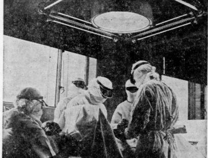
How ultraviolet radiation purifies the air in an operating room. eliminating danger of infection from bacteria in the atmosphere. Note the "sterilamp" in the ceiling, the long tube-like lights.
