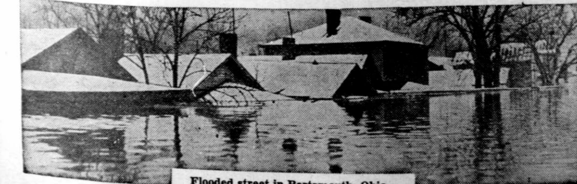
Flooded street in Portsmouth, Ohio.
