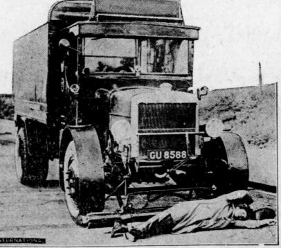
One of the most remarkable of the new safety devices is this appliance designed for the front of a motor car or truck to prevent victims from falling under the wheels of the vehicle before the driver can come to a full stop. The moment that the front of the car strikes a pedestrian, a roller is automatically dropped and made to revolve in a direction opposite to that of the wheels. The victim is thus propelled along the road until the driver has had time to stop his car.
