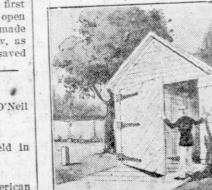
With Garage Doors of Unequal Width, as Shown, the Opening and Closing of Them in High Wind by One Person is Simple.
